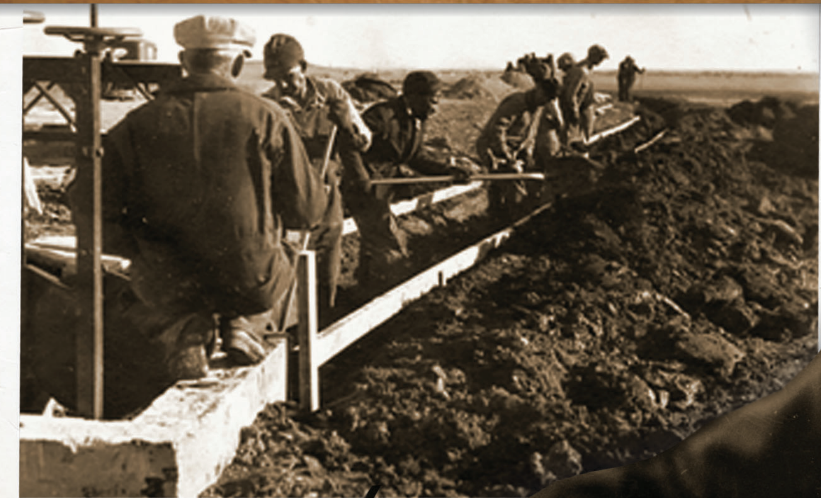
The CCC digging and forming-up a canal east of the main inlet box.
